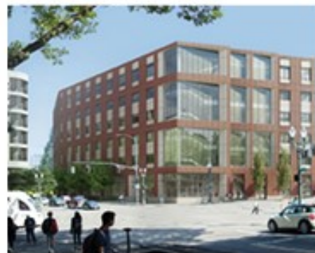
The New Lincoln High School building under construction at the current site
